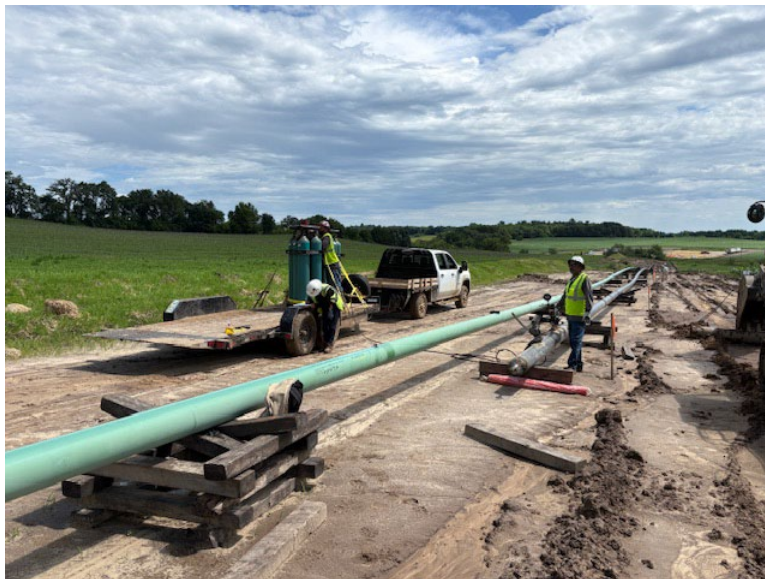
Facing northeast near MP 3.25, contractor setting up for nitrogen test on bore pipe
