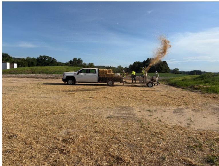
Facing north near MP 3.55, contractor mulching staging area
