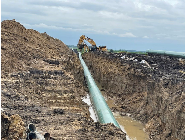
Facing south at MP 33.0, K&K lowering-in 36-inch-diameter mainline pipe south of 154th Street/County Road 80
