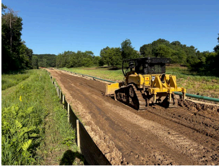
Facing northwest near MP 2.75, contractor working subgrade to help dry out right of way
