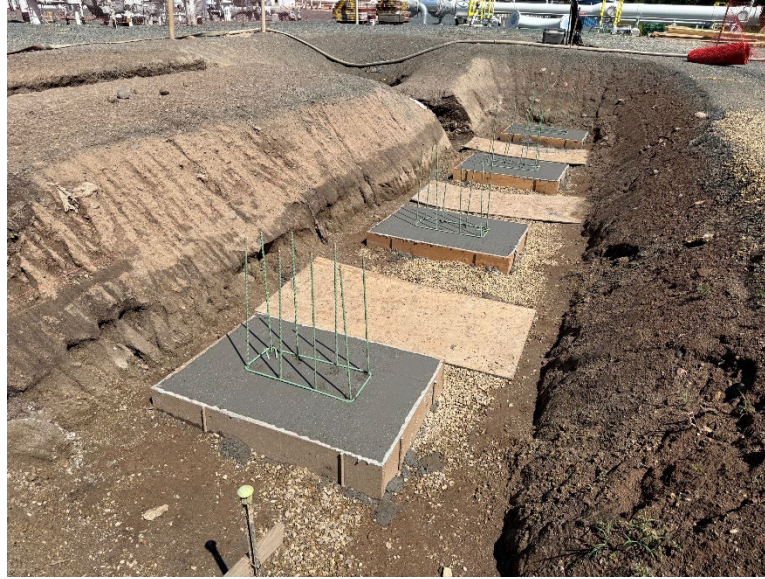
Facing east, view of the concrete forms poured in the Hugo compressor station near MP 0.1
