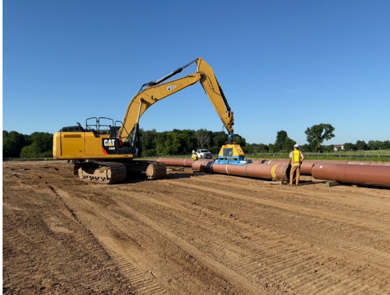
Facing west, Otis commences the stringing of the bore pipe near MP 0.1
