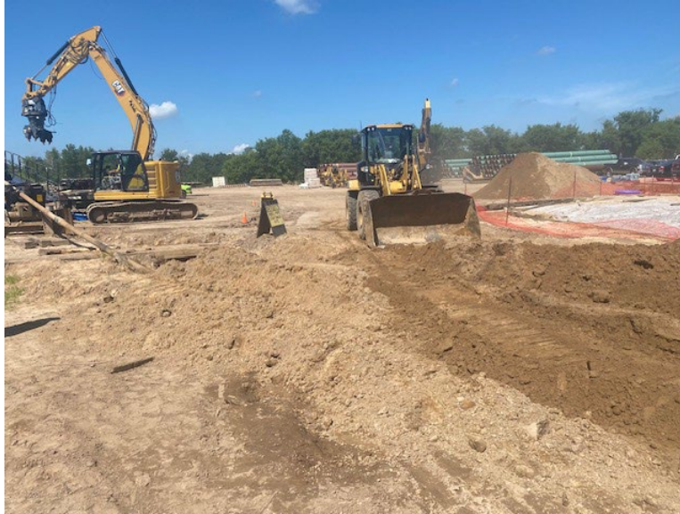
Facing west near MP 3.2, backfill completed at HDD P4-7 entry pit
