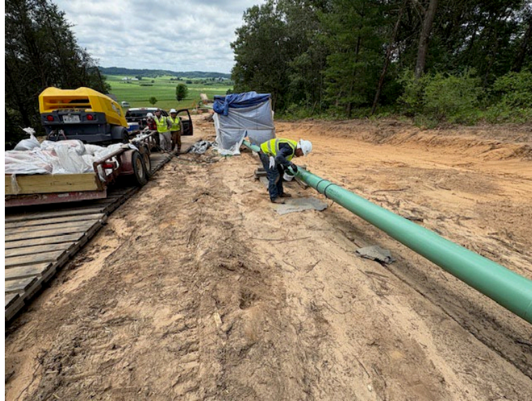
Facing west near MP 2.3, contractor sandblasting and coating branch line pipe
